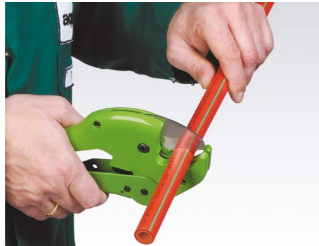
Cutting of the pipe
