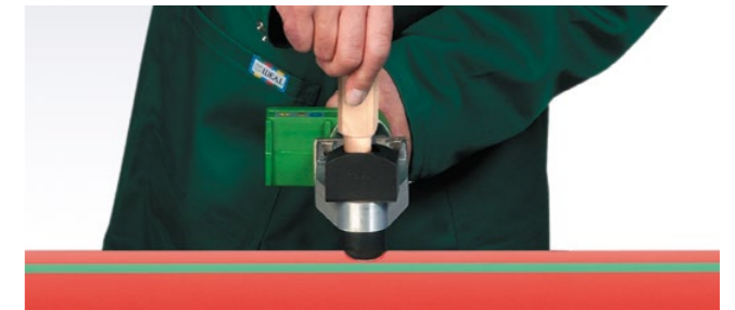
Heat-up of pipe ...
