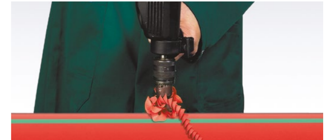
Drilling through the pipe wall
