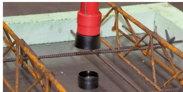
The upper part of the sprinkler outlet with pipe connection is attached to the base part of the sprinkler outlet.
