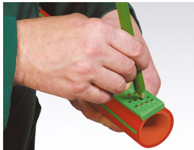
Marking of the welding depth
