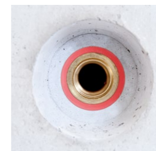
Illustration 3 finished sprinkler connection in the concrete ceiling
