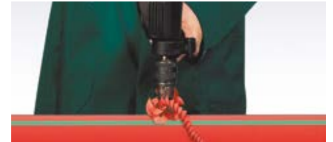
Drilling through the pipe wall
