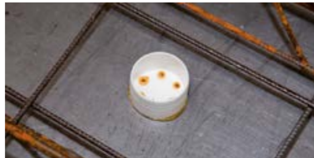
Base part of sprinkler outlet art. no. 3090000005 for concealed sprinklers. Attachment with hot-melt adhesive.
