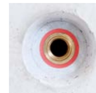
Illustration 3 finished sprinkler connection in the concrete ceiling
