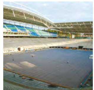
Undersoil pitch heating
