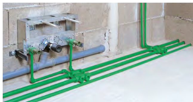
Floor distribution with distribution blocks
