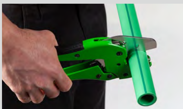
Cutting of the pipe
