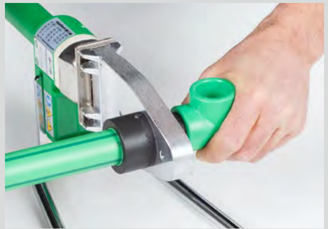
Heating-up of pipe and fitting
