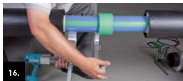
16. Open the clamping jaws of the pulling tool until the pulling tool can be removed sideways or downwards from the joint.
