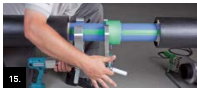
15. Loosen the clamping jaws on the moulded part side by unscrewing the fastening screw.
