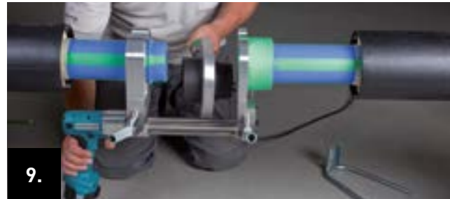
9. After the heating time has elapsed, move the pulling tool apart and remove the welding device between the pipe end and the moulded part.
