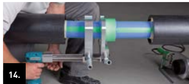
14. Move the pulling tool apart to be able to loosen the fastening screw of the moulded part clamping jaws.
