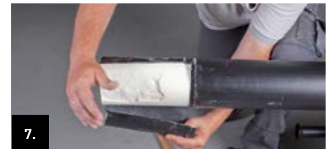
7. Cut off the end of the casing pipe and then mechanically remove the PUR insulation layer along the entire length of the insulation.
