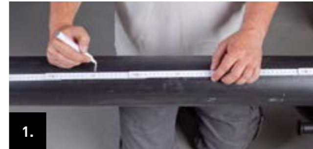
1. Measure the pipe length and mark it on the casing pipe.
