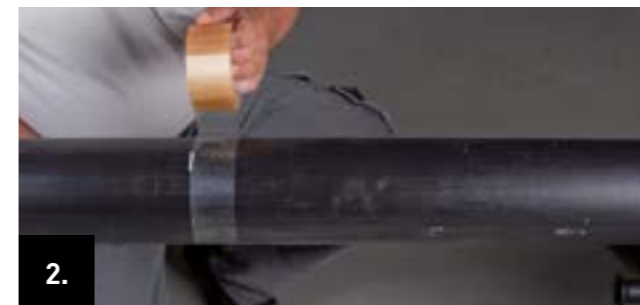
2. Mark the cutting line on the pipe circumference with adhesive tape.
