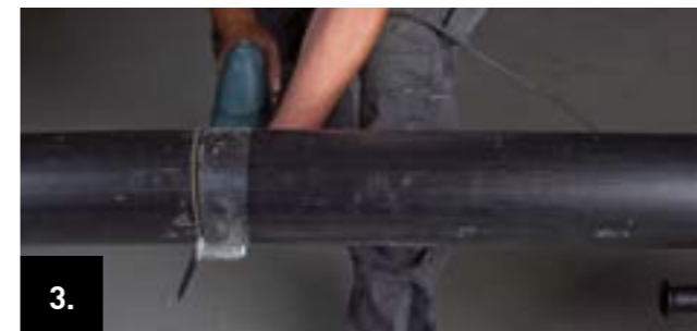
3. Cut the pipe along the cutting line using a standard tiger saw or foxtail equipped with a plastic saw blade.
