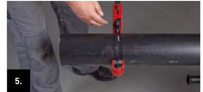
5. Cut through the entire circumference of the casing pipe with a pipe cutter up to the PUR insulation layer.
