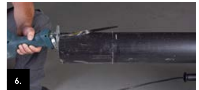
6. Cut the jacket down to the PUR insulation layer using a standard tiger saw or foxtail equipped with a plastic saw blade.
