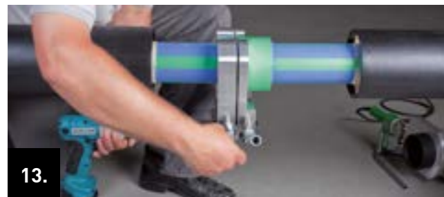
13. After the cooling time has elapsed, loosen the clamping jaws on the pipe side by unscrewing the fastening screw.
